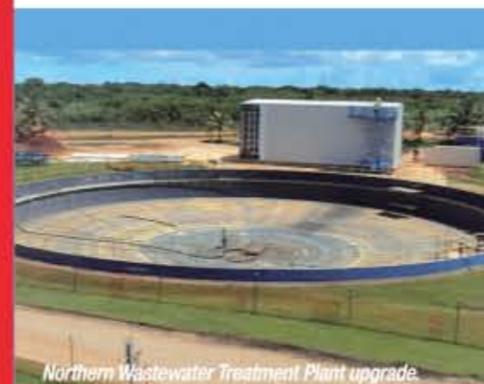
Northern Wastewater Treatment Plant upgrade.
