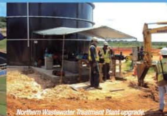
Northern Wastewater Treatment Plant upgrade.
