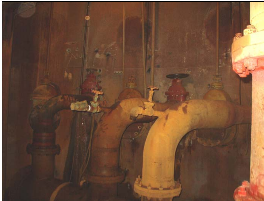
Collector well laterals, piped to manifold at bottom.
