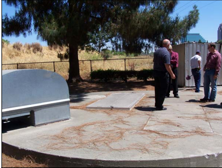
Concrete surface completion.
