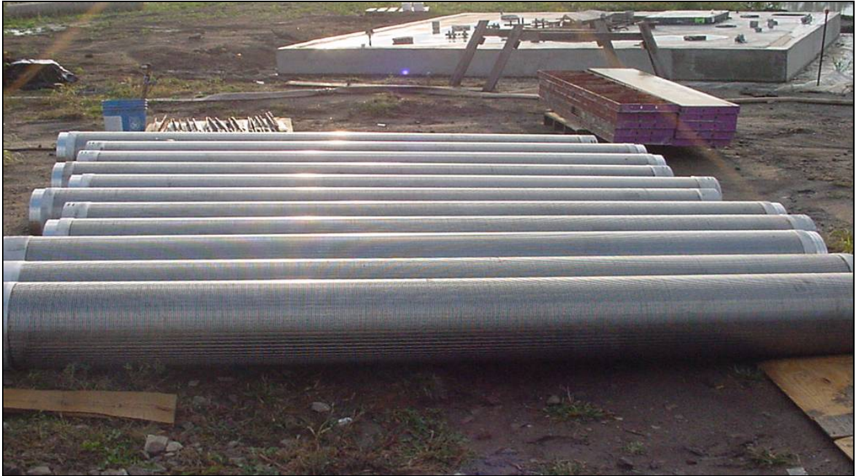
Collector well screens, prior to installation.
