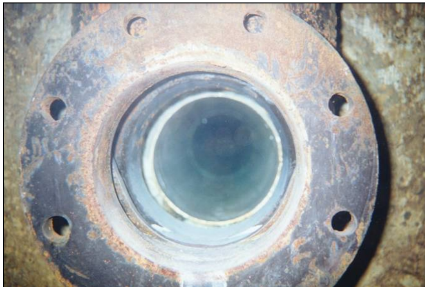
Collector well lateral, view from caisson.
