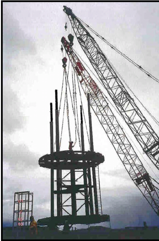
Figure 2-5 – Representative Photographs of Shaft Sinking Operations
