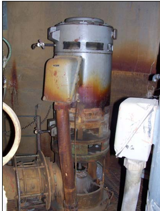
Collector well pump.
