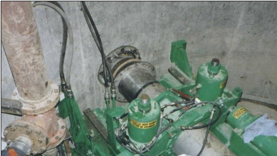
Jacking machine close-up.
