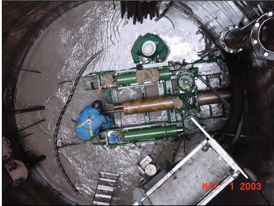
Jacking machine installing lateral from caisson.
