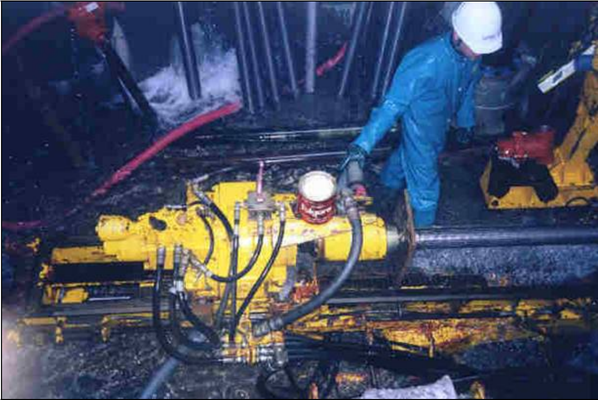
Jacking machine installing screen.
