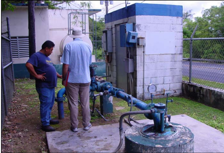
Figure 11-1 – Deep Well PS A-25
