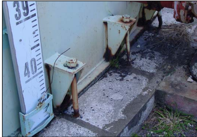
Picture shows extensive corrosion and total failure of hold down bolts near concrete base.
