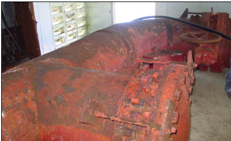
Figure 11-41 – Surface Corrosion and Pitting in Pipework in Effluent BPS
