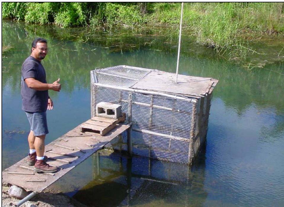
A general view of weir intake structure.
