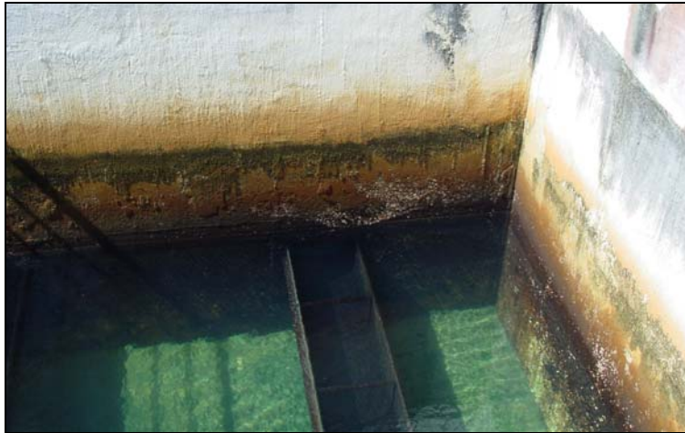
Filtration tank showing discolored but otherwise sound concrete.
