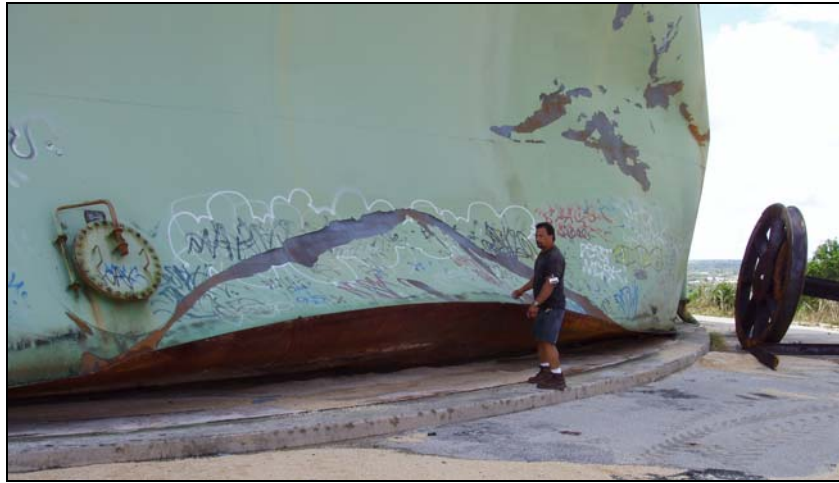
Figure 11-21 – Adjacent 2 mg Damaged Reservoir
