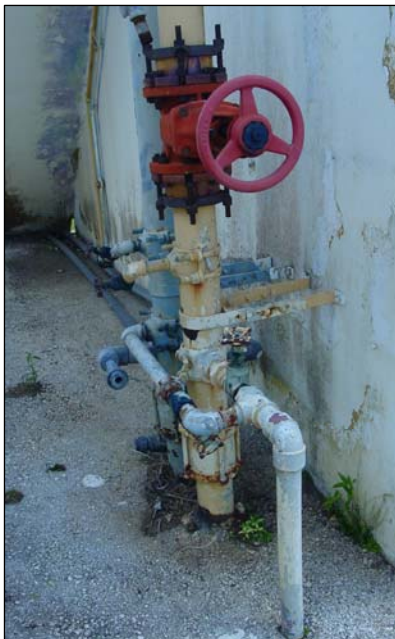
Figure 11-44 – Pipework H 2 S Corrosion at Centrifuge Building
