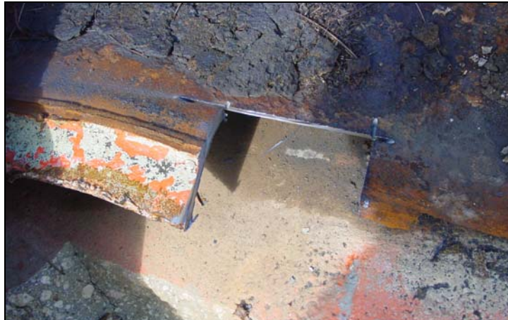
Figure 11-25 – Pitting Corrosion Damage on 1 mg Reservoir Wall
