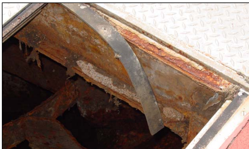
Figure 11-38 – Corroded Primary Support Beams for Aerator
