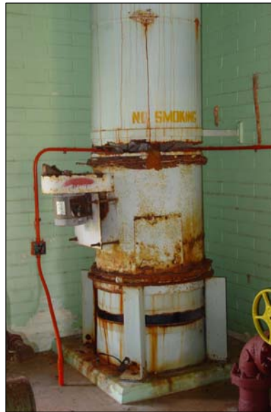
Figure 11-45 – Corrosion on Blower Ductwork at Heater/Digester Building
