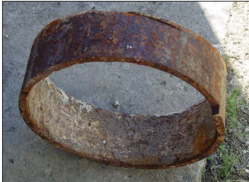
A ductile iron pipe segment showing relatively thin cement mortar lining.
