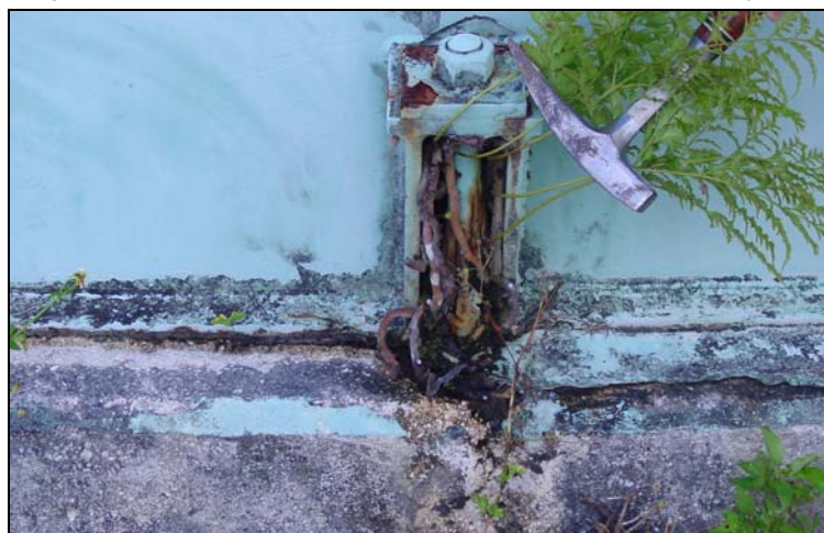
Figure 11-30 – Possible Earth Connection for Under-Floor CP System
