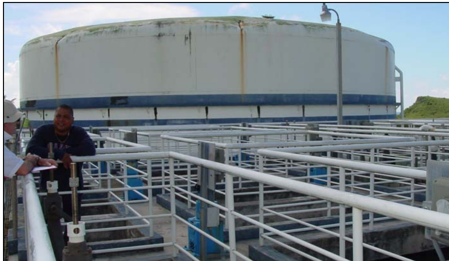
General view of Ugum WTP including storm damaged clear water tank.
