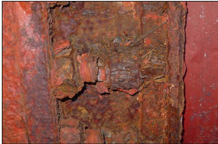
Figure 11-42 – Close-up of Failed Fastener from Figure 11-41
