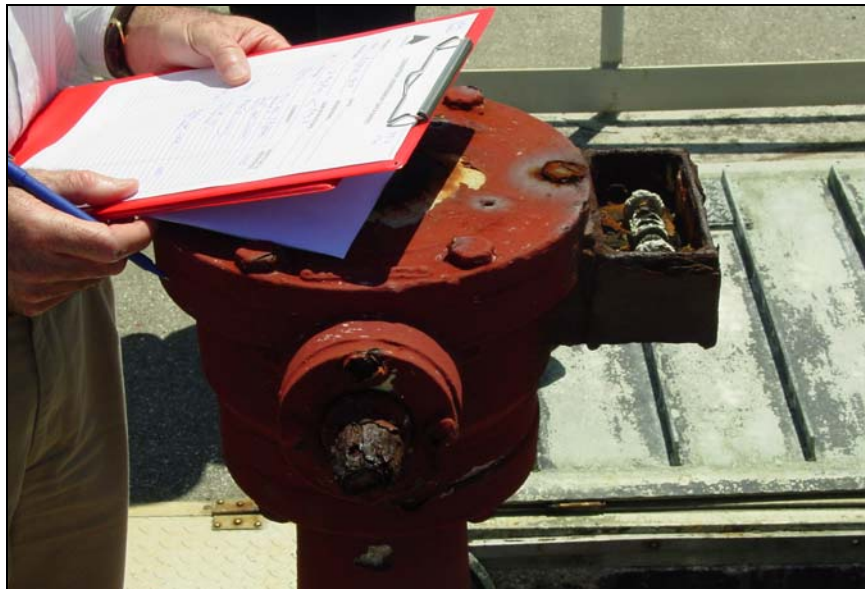
Figure 11-35 – Corrosion of Penstock Gate Valve
