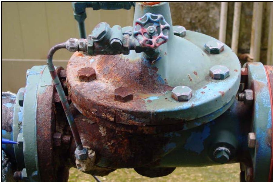
Figure 11-2 – Surface Corrosion on Pipework Flange
