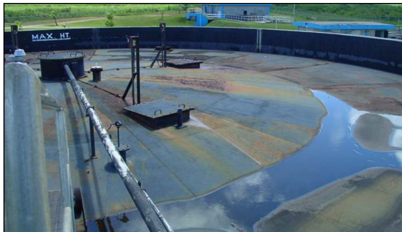
Figure 11-47 – Empty Clarifier Showing Bolt-on Sacrificial CP Anodes
