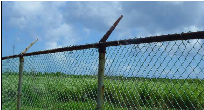
Figure 11-48 – Corrosion of Perimeter Fence
