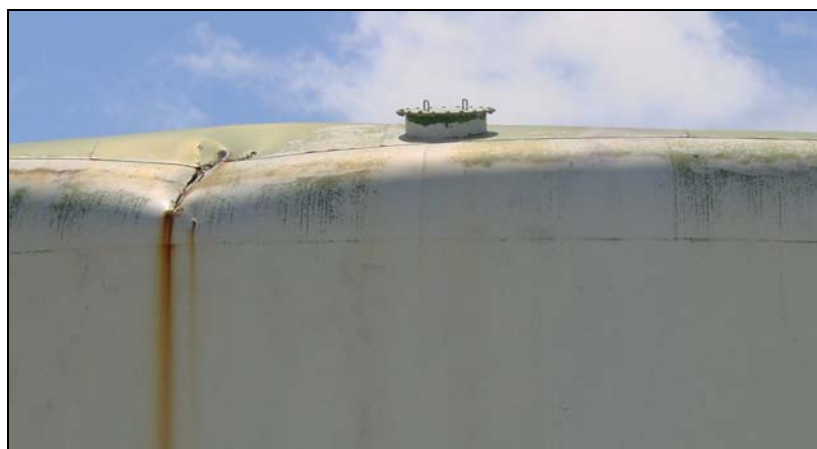
Figure 11-15 – Close-up of Partially Collapsed Roof
