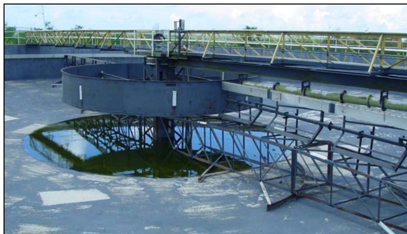
Figure 11-47 – Empty Clarifier Showing Bolt-on Sacrificial CP Anodes
