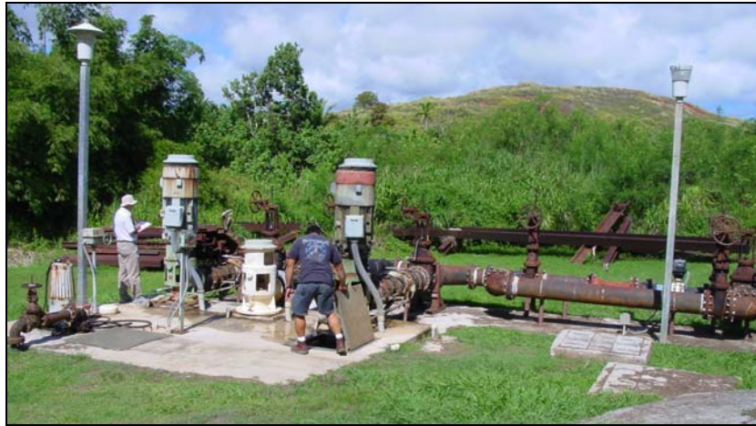
A view of the two pumps at the intake works
