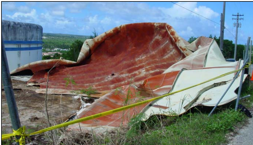
Figure 11-20 – Part of Walls and Roof of Collapsed Reservoir
