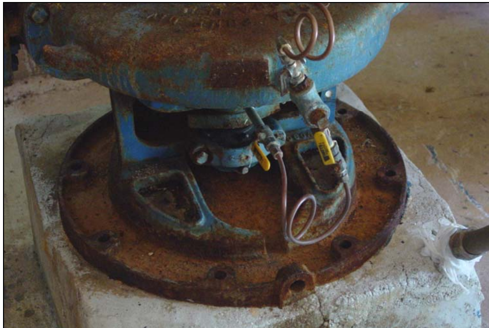
Pump base plate not bolted to concrete foundation.
