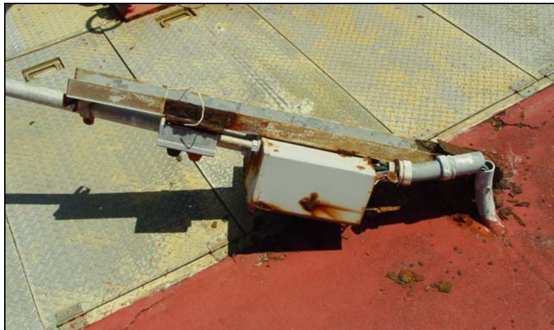
Figure 11-37 – Failed Power Supply Support to Aerator
