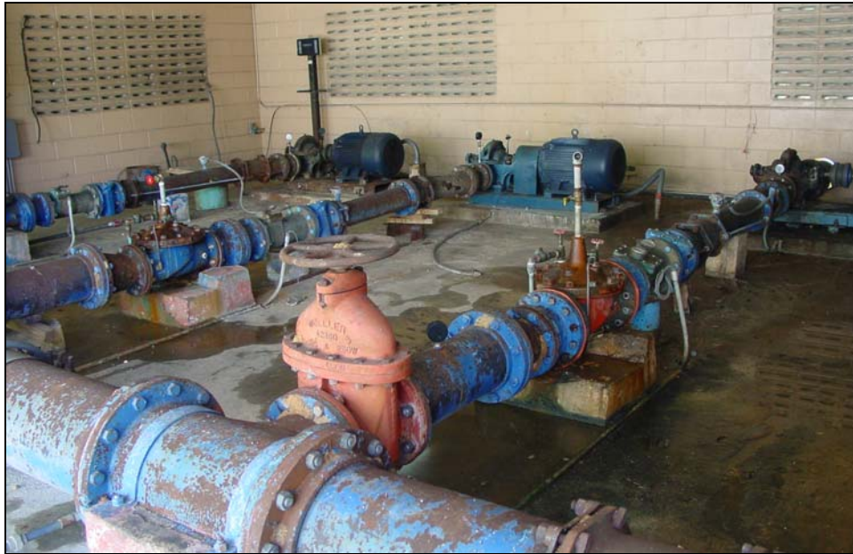
Figure 11-4 – Internal View of PS Pipe Layout
