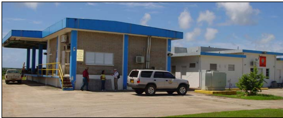
Figure 11-43 – General View of Chlorination, Laboratory and Operational Buildings
