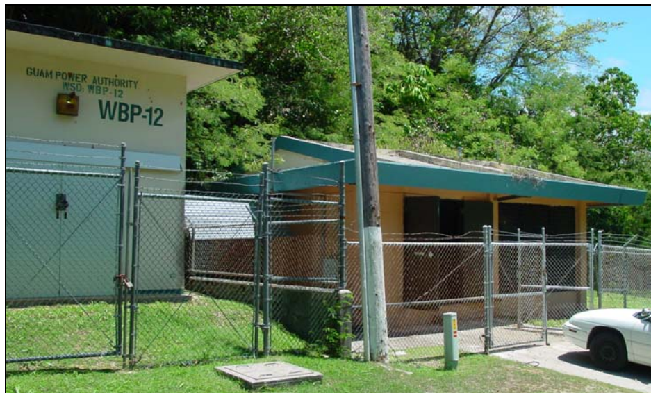
An external view of Brigade Bay PS.
