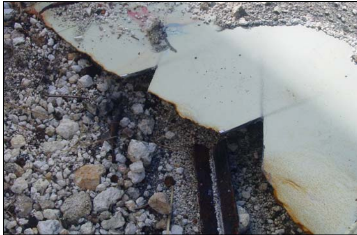
Figure 11-22 –Collapsed Reservoir Wall Showing Positions of Sample Removed for Analysis
