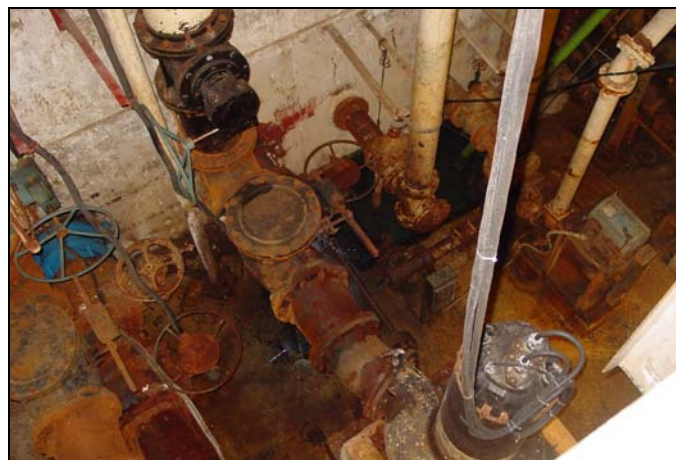
Figure 11-32 – Pump Arrangement Inside Dry Well
