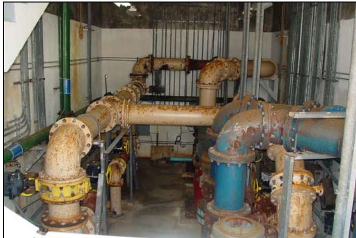
Figure 11-14 – Pipe Gallery Under Control Room
