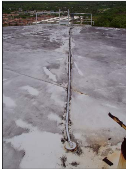
Part of conduit used for (non-operational) cathodic protection.
