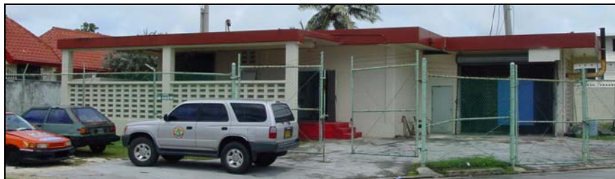
Figure 11-31 – External View of Hagatna STP
