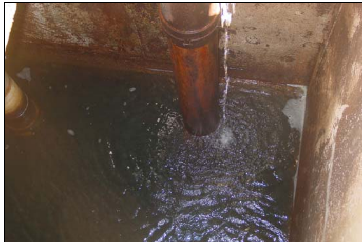
Note good condition of concrete.
