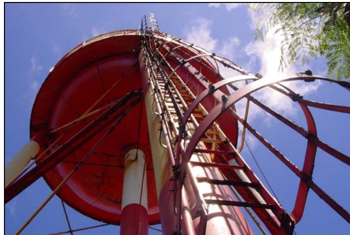
Picture shows view of corroded ladder and supports on high level tank.
